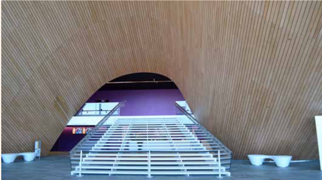
Kilden cultural center in Norway. Billowing oak wall treated with ES/VFR flame retardant coating to B s1 d0.
