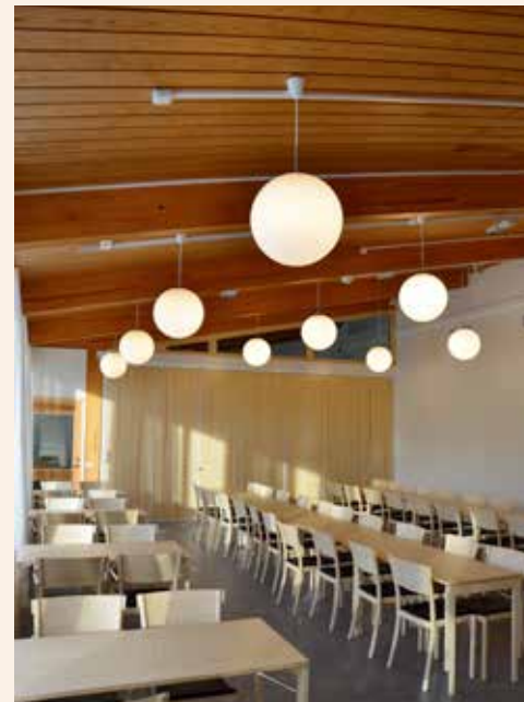
Church in Sweden. Wooden ceilings treated with ES/VFR flame retardant coating to B s1 d0.
