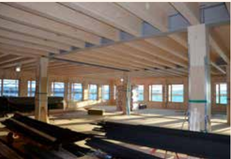
Kongsvinger Festing in Norway. Internal wood treated with HW01 intumescent paint to EI30.
